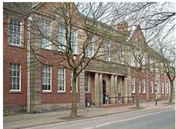
The former technical college, Stoke, now part of Staffordshire University.
